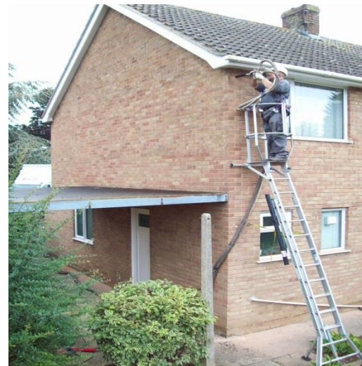
Pumping insulation into cavity
