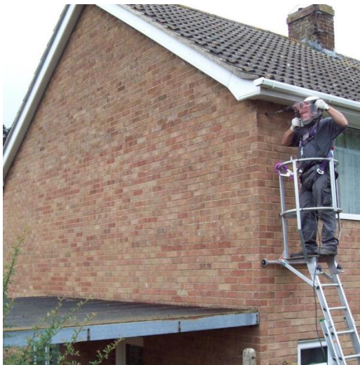
Drilling hole ahead of cavity fill
