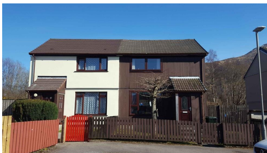
Left – EWI Installed Right – without EWI
